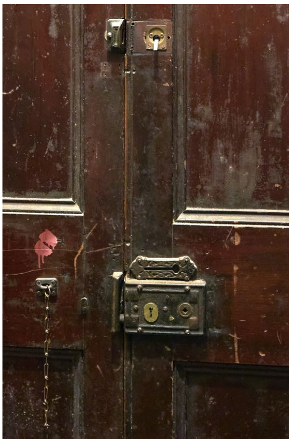
Figure 50: Rim Lock and hardware to south door
