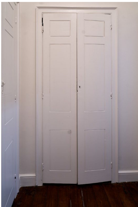
Figure 56: Cedar cupboards painted white in room G06
