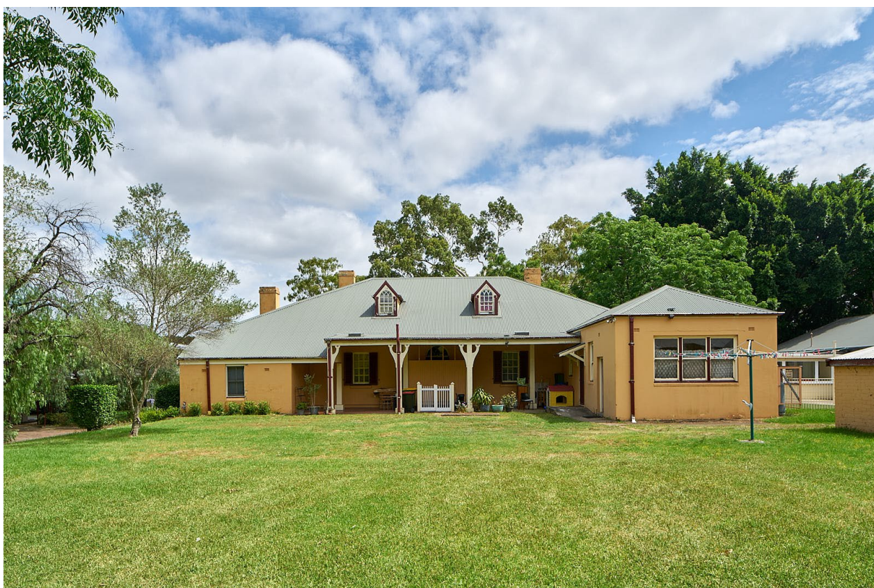
Figure 81: The south elevation showing the dormer windows to the attic.
