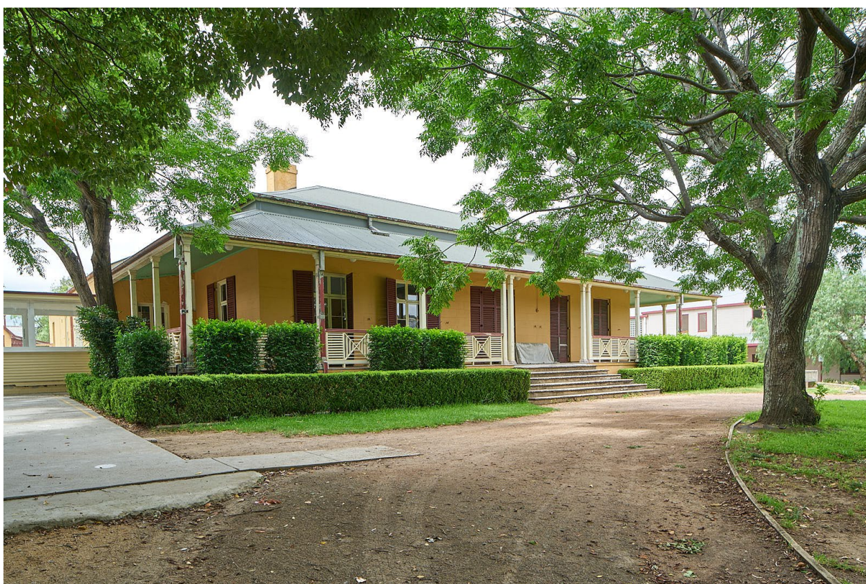
Figure 75: View from the carriage drive approaching from the northeast. 2023.
