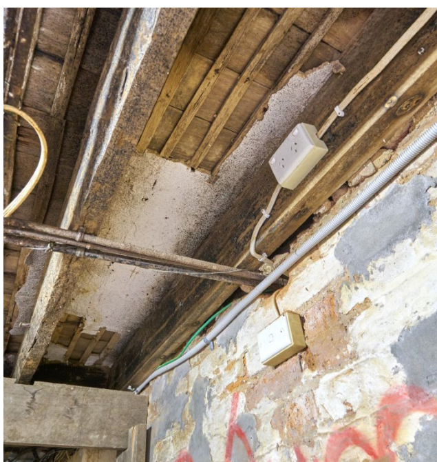
Figure 22: Evidence of plaster on the cellar ceiling
