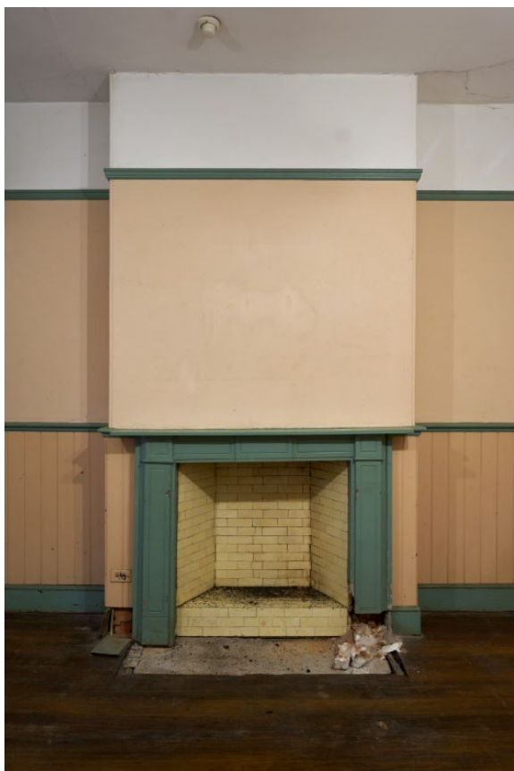
Figure 52: Chimney piece in room G05
