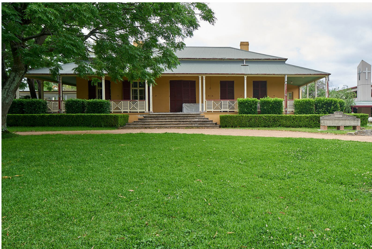
Figure 76: The north façade 2023.
