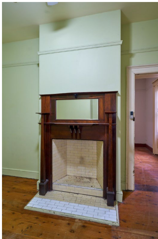
Figure 55: Chimney piece in room G11
