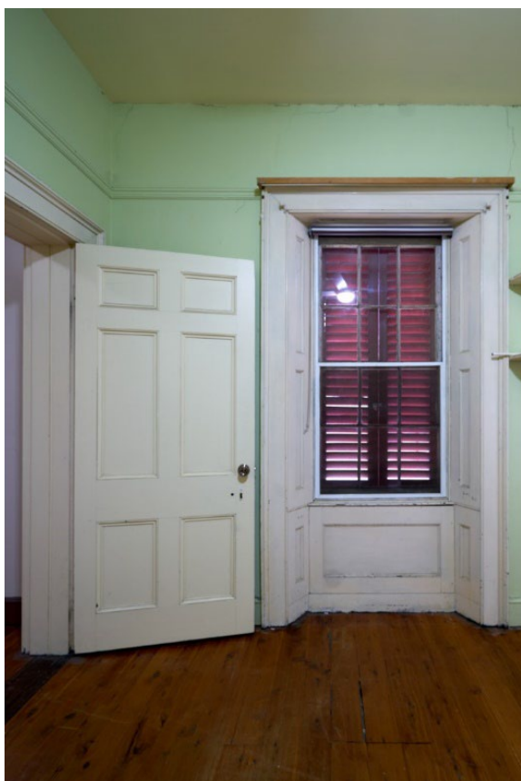
Figure 58: Window and door joinery in room G11
