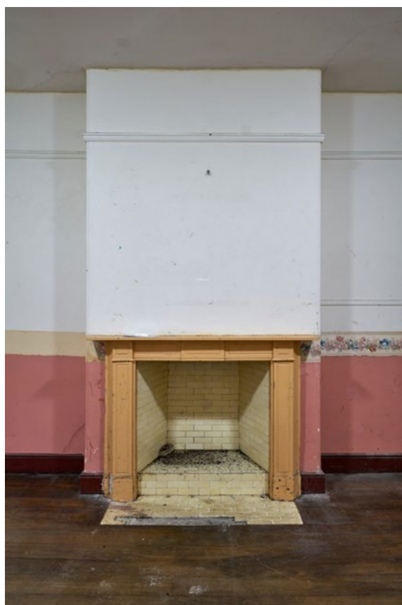
Figure 53: Chimney piece in room G10
