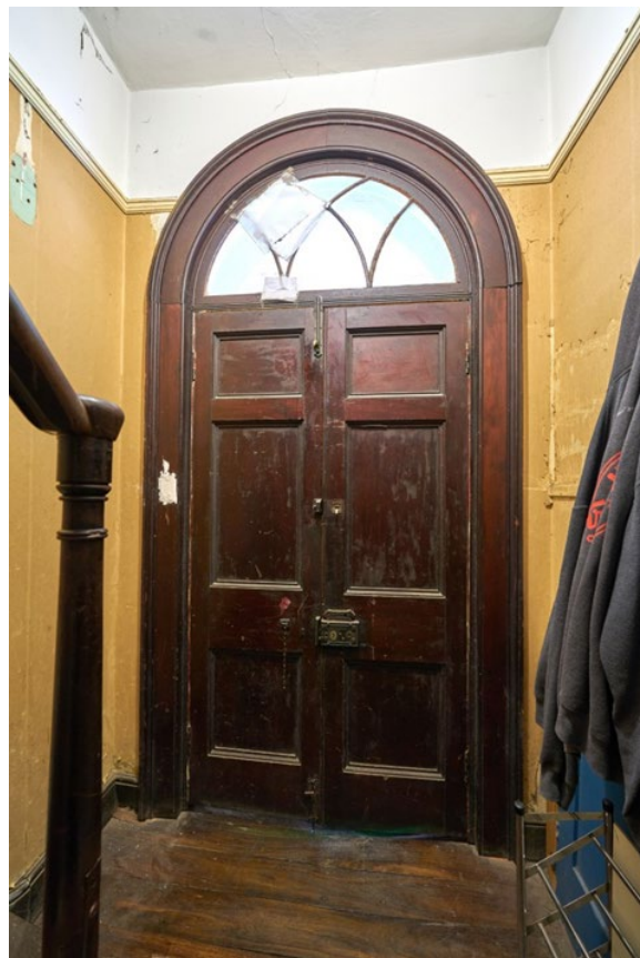
Figure 25: Double doors to the south of the hall.
