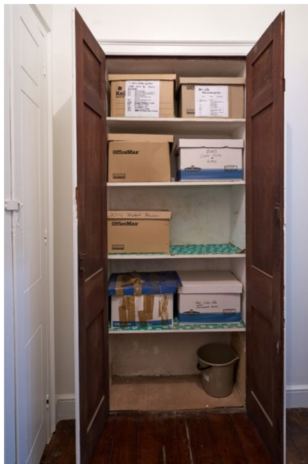
Figure 27: Interior of cupboard showing original timber
