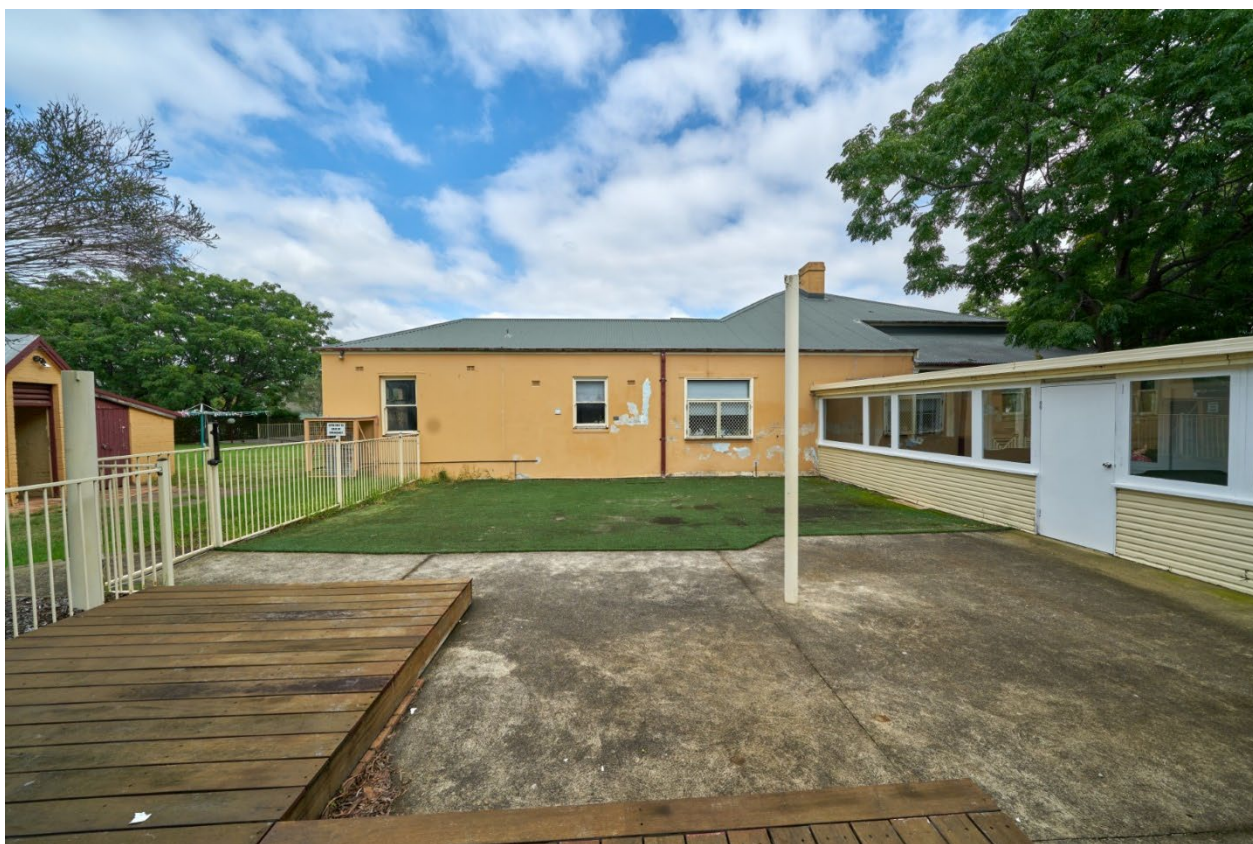
Figure 83: The eastern elevation showing the link to the right of the image. 2024.
