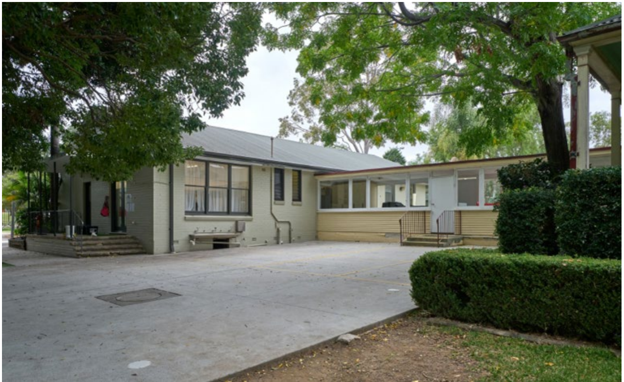
Figure 77: Ebsworth House from the North. The corner of The Homestead can be seen on the right. JPA&D 2024.
