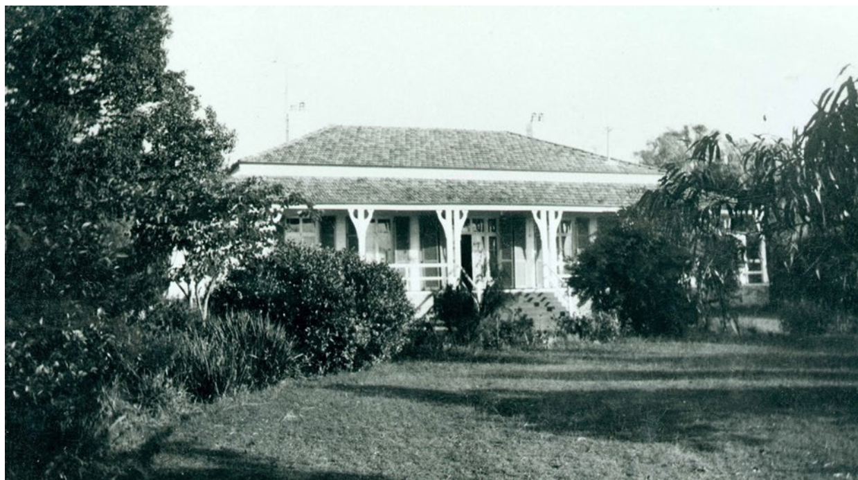
Figure:14 North façade of the Homestead in 1960. Canterbury Bankstown Library PH-0000389 1960
