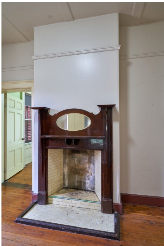
Figure 54: Chimney piece in room G12
