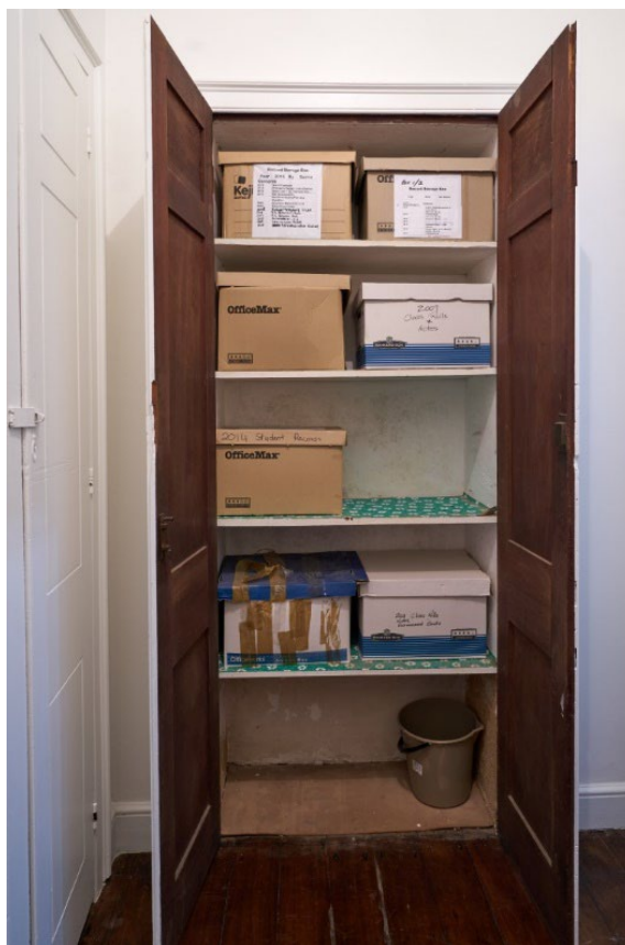
Figure 57: Interior of cupboard showing cedar joinery.
