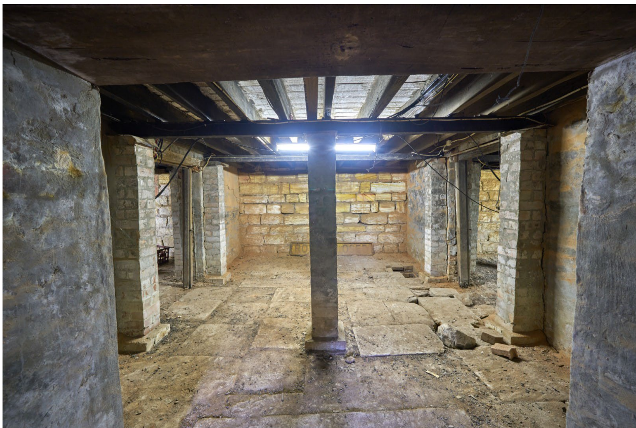
Figure 21: The Basement looking north from the entrance showing stone flagged floor and stone north wall.
