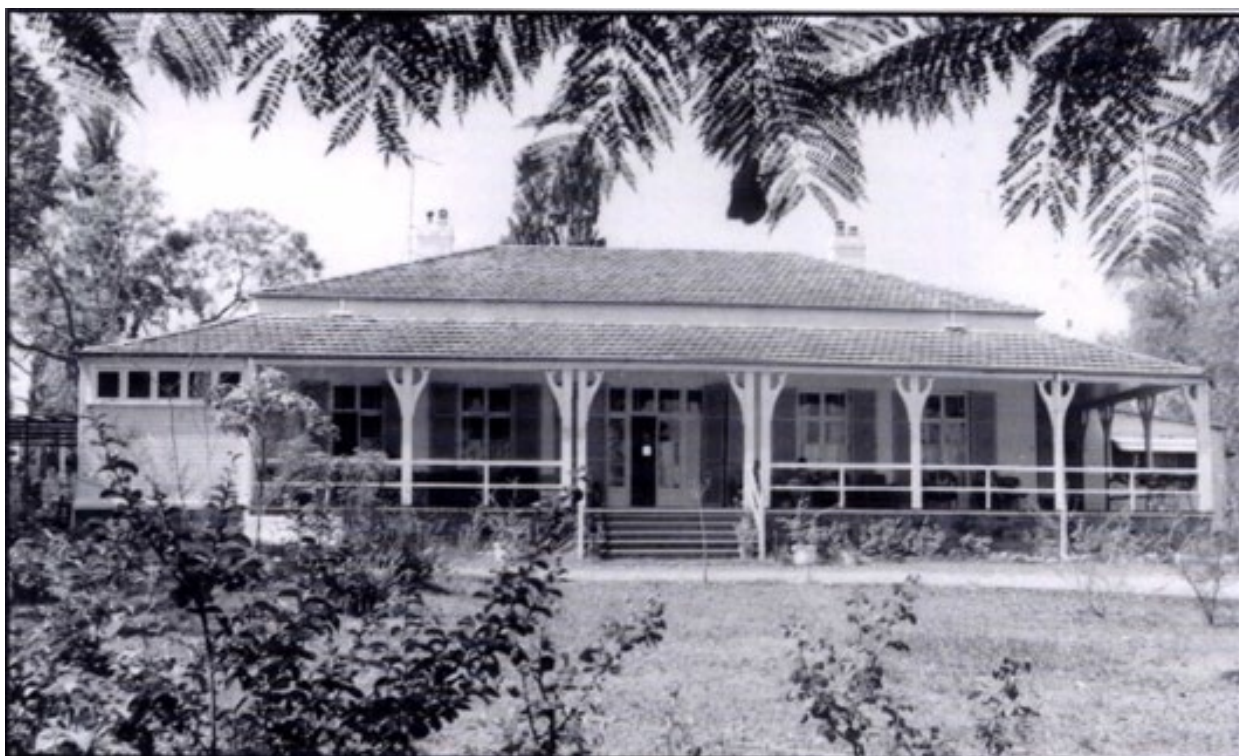
Figure 28: The north elevation of the homestead c. 1960 showing the infill to the verandah, changes to the verandah and an extension to the west of the building.
