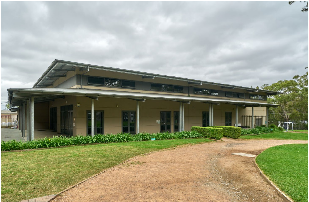
Figure 8: Gymnasium built 2010 under the Government Building Education Revolution (BER) program. JPA&D 2024.
