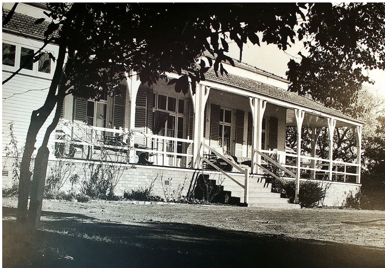
Figure 12: View of the front verandah c1960. Note the brick wall to the verandah, concrete steps, horizontal balustrade and infill to the northeast corner. Canterbury Bankstown LibraryPH-0001940
